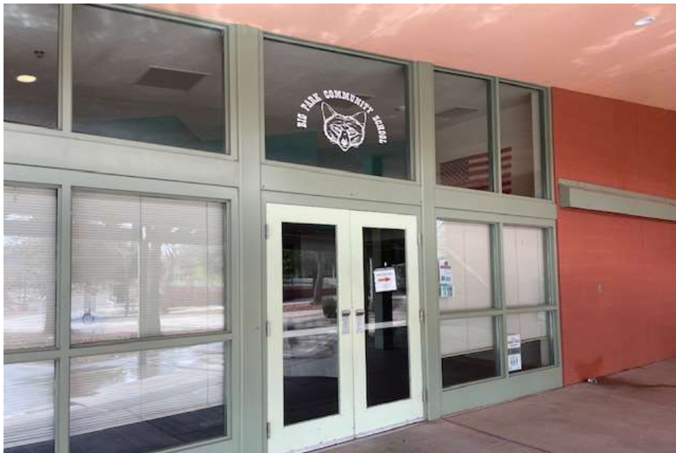
Subject building entrance
