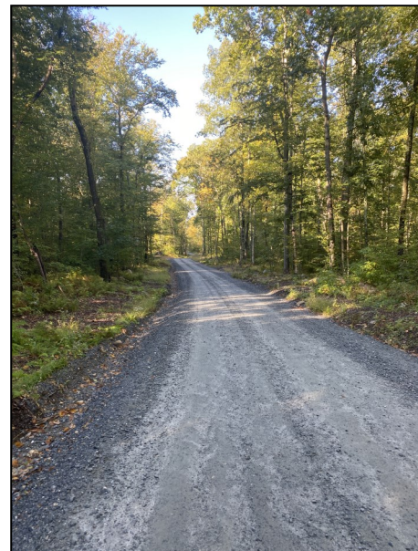
Ackley Road after the construction.
